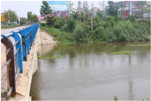
跨河桥梁边坡预制块防护
