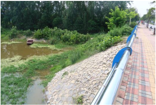
跨河桥梁边坡预制块防护
